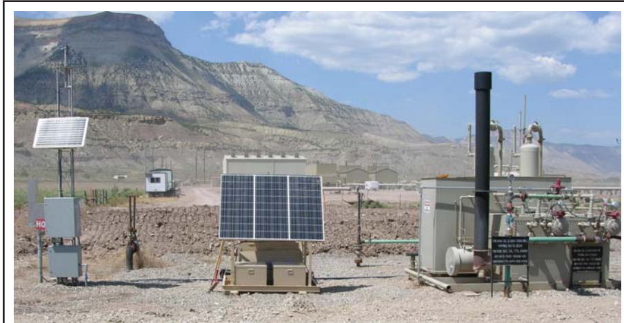
The AirMax™ controller from J&J Solutions can be powered by wind, a solar panel or a battery pack to operate a gas compressor control system as well as glycol pumps, separator dumps, motor valves, plunger lift, diaphragm pumps and other equipment, saving fuel gas and eliminating emissions.
